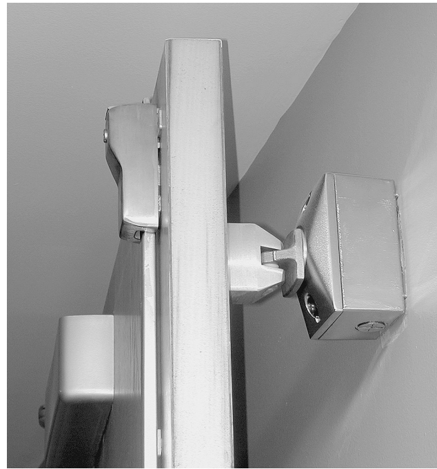
Exhibit 8.8 Hold-open mechanism on automatic-closing door.
