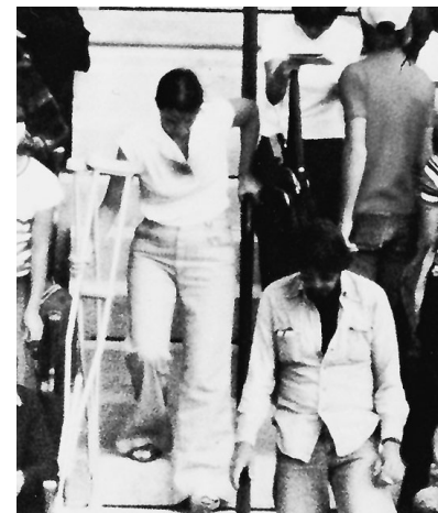
Exhibit 12/13.20 Intensive use of stadium aisle stair, 48 in. (1220 mm) wide with center handrail. (Photograph courtesy of Jake Pauls)
