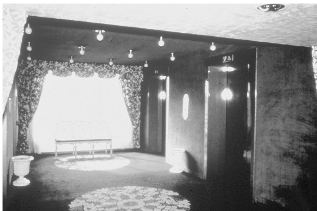
Exhibit 10.4 Elevator lobby with carpetlike textile wall and ceiling finish material.
