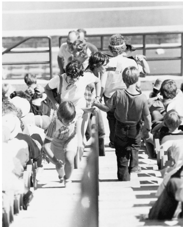
Exhibit 12/13.21 Intensive use of stadium handrail, approximately 34 in. (865 mm) high, at center of 48 in. (1220 mm) wide aisle stair. (Photograph courtesy of Jake Pauls)
