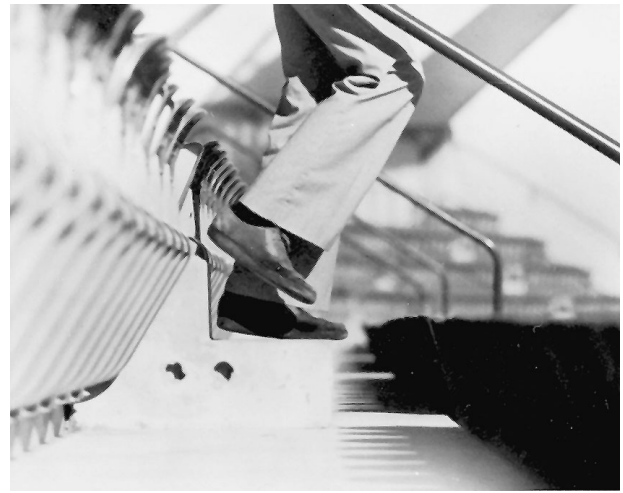
Exhibit 12/13.23 Side view of aisle stair with uniform tread depth of 11 in. (280 mm). (Photograph courtesy of Jake Pauls)
