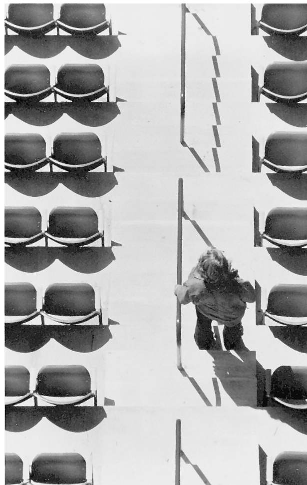
Exhibit 12/13.22 Overhead view of 48 in. (1220 mm) wide aisle stair with center handrail. (Photograph courtesy of Jake Pauls)
