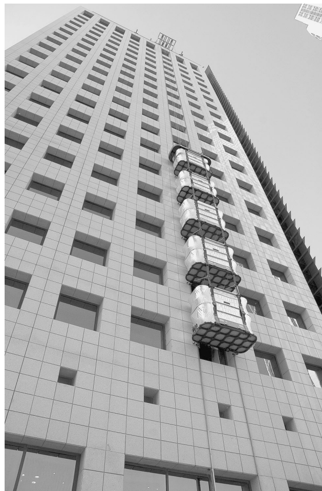
Exhibit C.4 Roof-supported platform rescue system with multiple platforms as installed on high-rise building. (Photo courtesy of Escape Rescue Systems, Ltd.)
