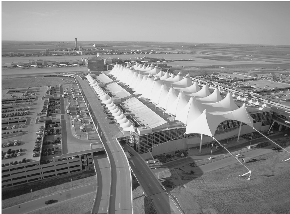
Exhibit 11.7 Example of a tensioned-membrane structure: Denver International Airport. (Photo courtesy of the Denver International Airport)
