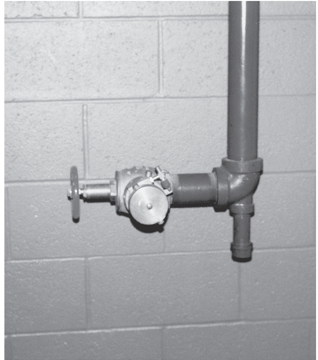
EXHIBIT 3.1 Class I Standpipe System
