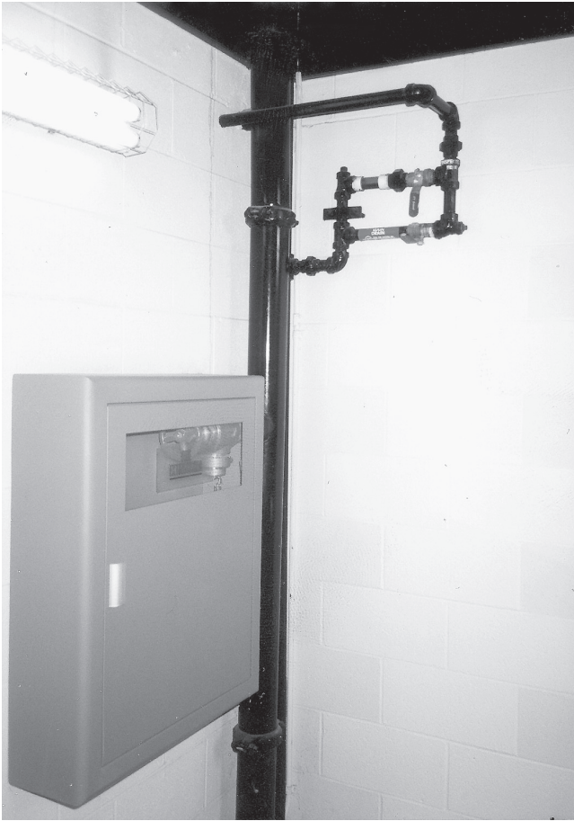
EXHIBIT 3.2 Class III Standpipe System
