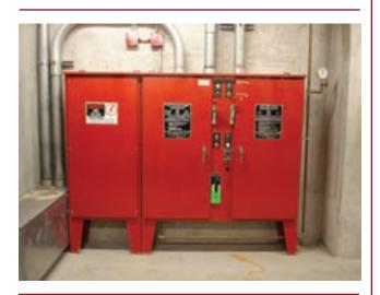
**EXHIBIT 695.6** Listed Fire Pump Controller and Power Transfer Switch.
