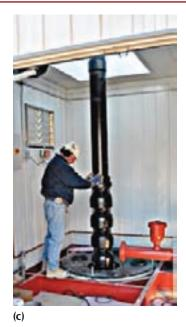
EXHIBIT II.7.3 Vertical Turbine Fire Pump Installation. (a) Unloading a vertical turbine pump. (b) Lowering a vertical turbine fire pump through a fire pump house roof hatch. (c) Lowering a vertical turbine fire pump into a wet pit. (d) Installing a motor on a vertical turbine fire pump. (Chris Gray, Fire Spec Sprinkler Supply Co.)
