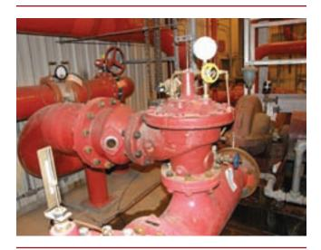
In this case, a pressure relief valve (see Exhibit II.4.16) is needed if the fire protection system components are rated at 175 psi (912.1 bar). A pressure relief valve is not required if the fire protection system components are rated for 200 psi (13.8 bar) or higher.
