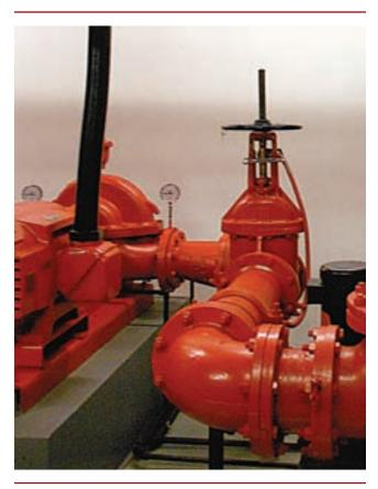
**EXHIBIT II.4.10** Pump Suction Elbow Installed in the Incorrect Plane.
