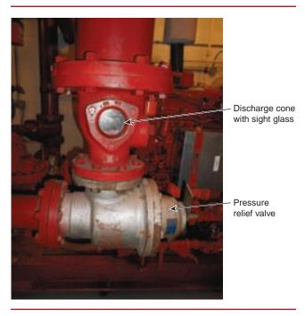
**EXHIBIT II.6.10** Pressure Relief Valve Piped Back to Suction.(Courtesy of Peerless Pump Fire Segment)
