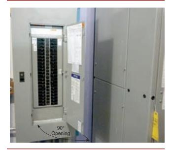
EXHIBIT II.10.8 Illustration of the Depth of Working Space Which Must Be Sufficient to Allow a Full 90 Degree Opening of Equipment Doors for a Safe Working Approach.
