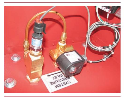
**EXHIBIT II.12.16** Pressure Transducer Mounted Inside of Controller.
