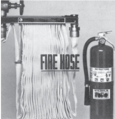
FIGURE A.3.3.19.4 Semiautomatic Hose Rack Assembly.
