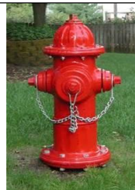
Private Service Main, less than 500 GPM. 6" main
