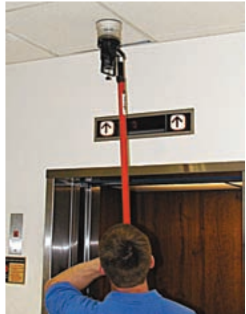
Functional Testing of Smoke Detector. (Courtesy of Jeffrey Moore, P.E., Hughes Associates, Inc., Baltimore, MD)
