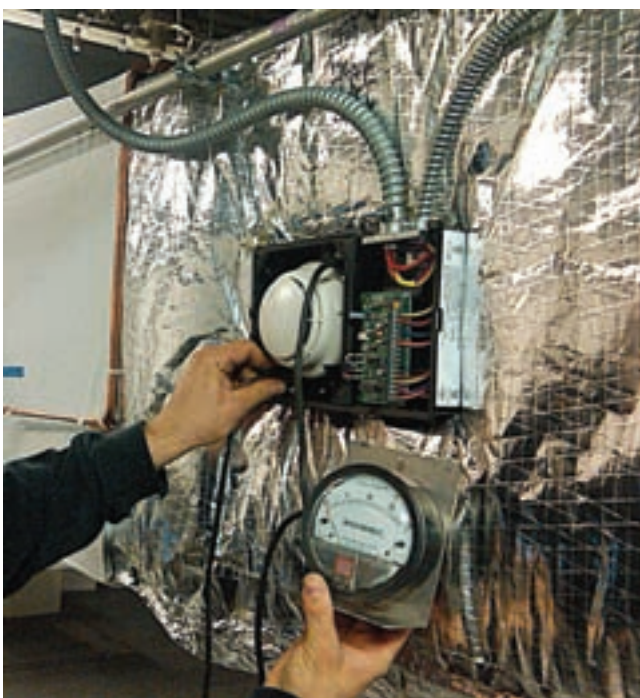
Duct Detector Installation Being Tested with a Manometer. (Courtesy of Warren Olsen, FSDI, Elgin, IL)
