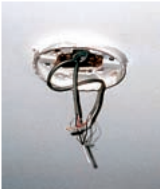
Installation with Missing Detector. (Courtesy of Jeffrey Moore, P.E., Hughes Associates, Inc., Baltimore, MD)
