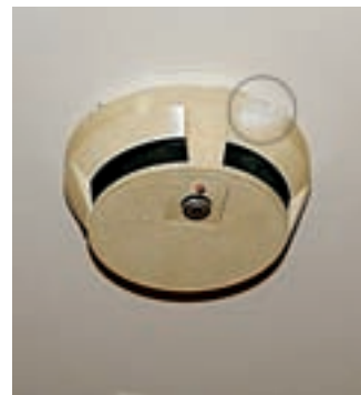
Combination Smoke and Heat Detector. (Courtesy of Jeffrey Moore, P.E., Hughes Associates, Inc., Baltimore, MD)
