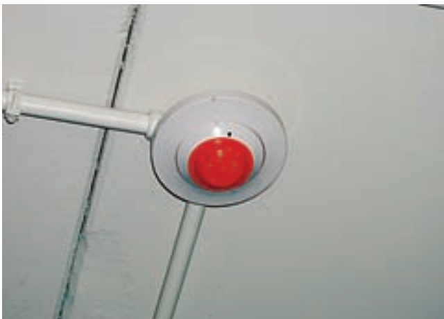
Smoke Detector with Cover Not Removed after Construction. (Courtesy of Jeffrey Moore, P.E., Hughes Associates, Inc., Baltimore, MD)
