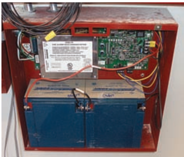
Visual Inspection of Batteries. (Courtesy of Jeffrey Moore, P.E., Hughes Associates, Inc., Baltimore, MD)
