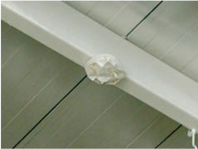
Heat Detector Covered with Tape. (Courtesy of Jeffrey Moore, P.E., Hughes Associates, Inc., Baltimore, MD)
