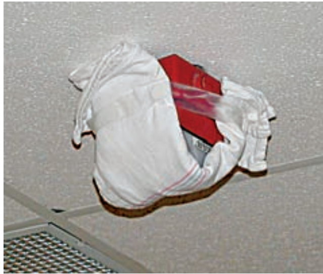
Evidence of Appliance Tampering. (Courtesy of Jeffrey Moore, P.E., Hughes Associates, Inc., Baltimore, MD)
