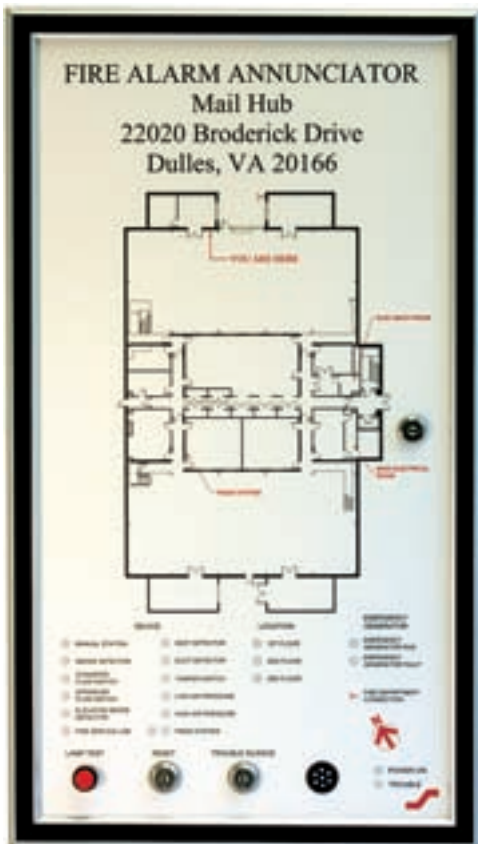
Typical Graphic Fire Alarm Annunciator. (Source: Space Age Electronics, Inc., Sterling, MA)
