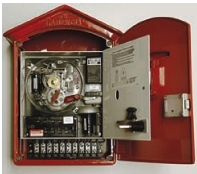
Inside View of Master Box. (Source: R. B. Allen Co., North Hampton, NH)
