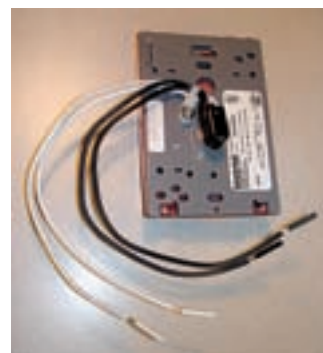
Initiating Device Showing Duplicate Leads. (Source: Edwards, Bradenton, FL)
