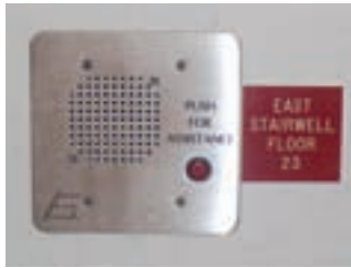
Area of Refuge Station Used for Emergency Communications. (Courtesy of Jeffrey Moore, P.E., Hughes Associates, Inc., Baltimore, MD)
