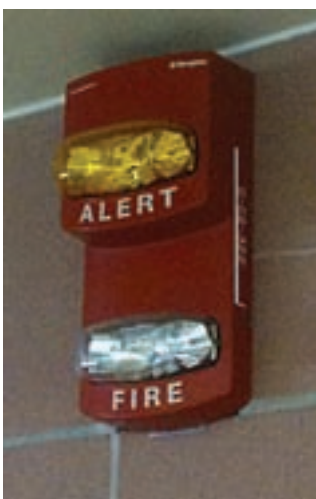
Combination Fire/Alert Visible Notification Appliance.
