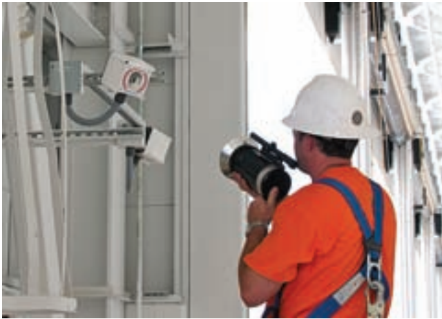
Testing the Response of a Flame Detector. (Courtesy of Jeffrey Moore, P.E., Hughes Associates, Inc., Baltimore, MD)
