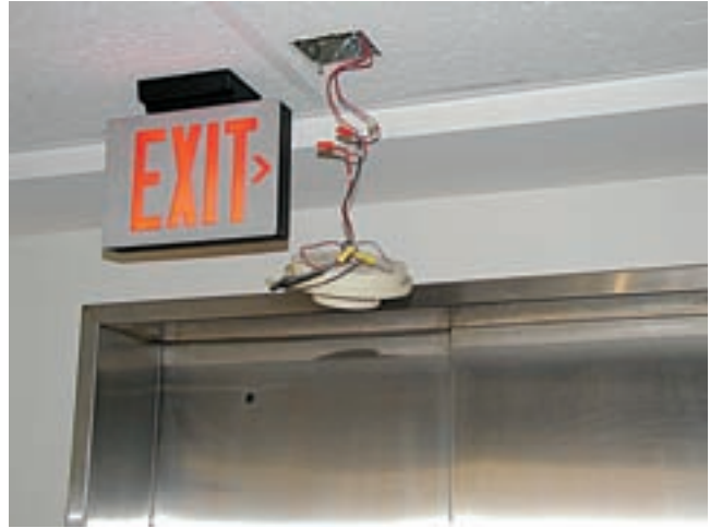
Smoke Detector Improperly Secured. (Courtesy of Jeffrey Moore, P.E., Hughes Associates, Inc., Baltimore, MD)
