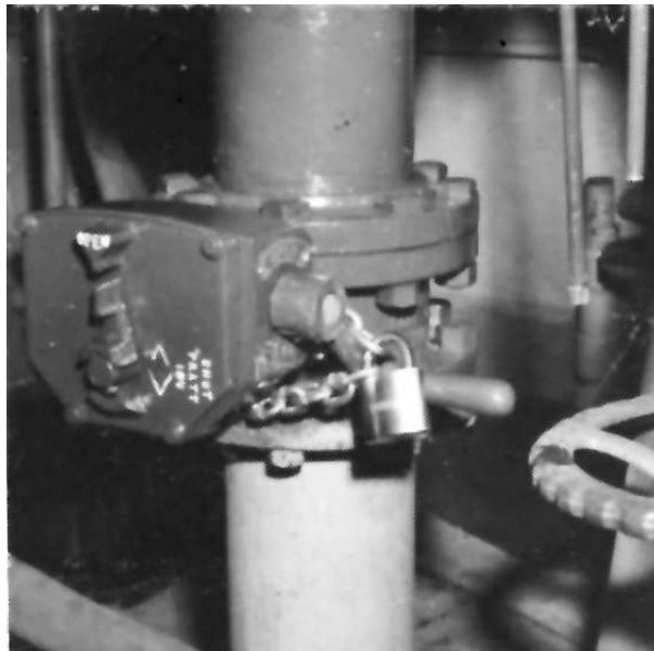
Fig. 5. Indicating butterfly valve (IBV).
