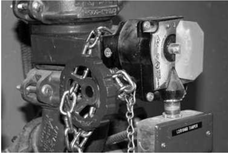
Fig. 6. Indicating butterfly valve (IBV) with handwheel.
