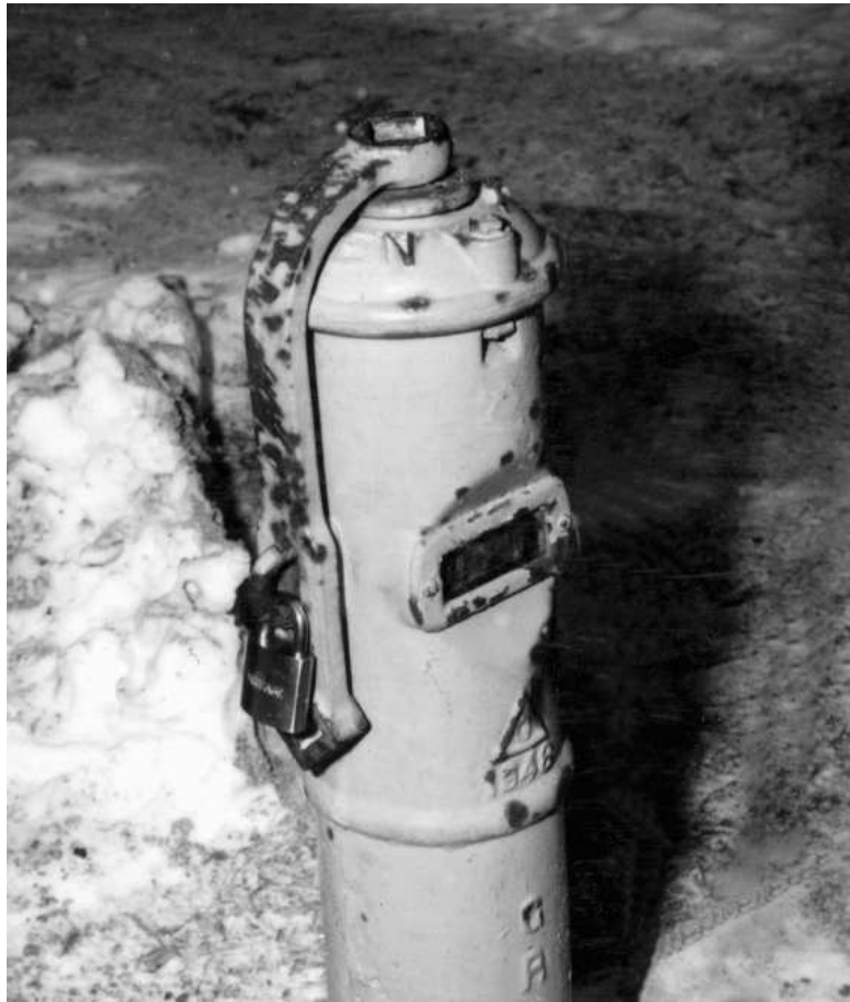
Fig.1. Post indicator valve
