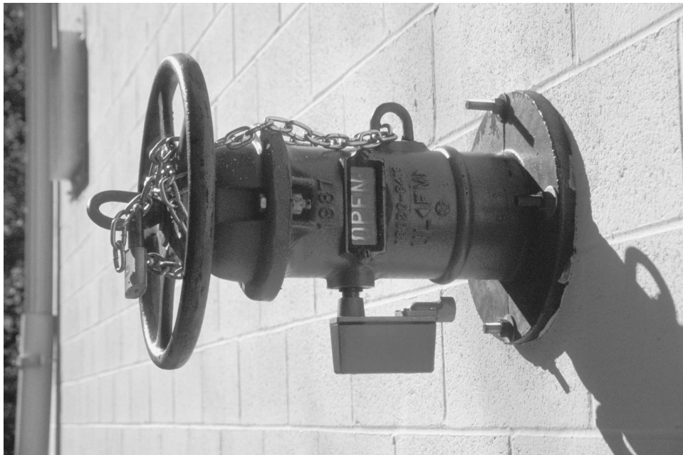
Fig. 3. Wall post indicator valve with handwheel eye bolt.
