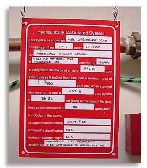
This nameplate is typical of the style that should be found on a hydraulically calculated sprinkler system.
