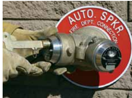
Locking 2 1/2" Plug with Knox Keywrench
