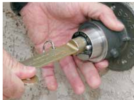
Locking 1 1/2" FDC Plug with Knox Keywrench
