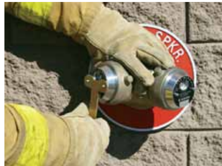
Loosening 2 1/2" Plug with Knox Keywrench
